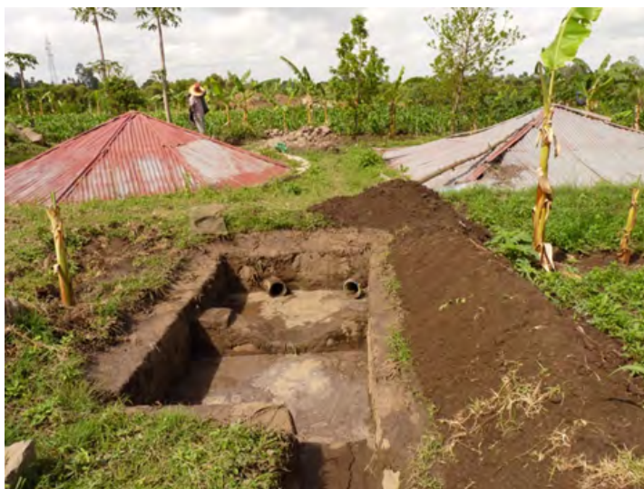
Figure 2: Farm ponds in Halaba special woreda (Central Rift valley of Ethiopia) with sediment trap in front.
