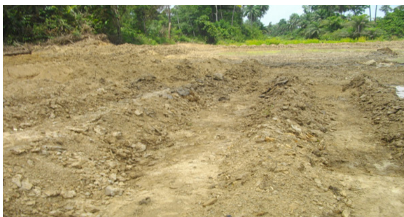
Figure 2: Making of windrows during bioremediation of polluted soil in Ikarama community, Bayelsa State.
