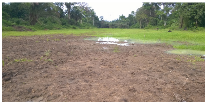
Figure 3: Levelling of windrows after bioremediation has been completed and emergence of green grasses as evidence of a successful bioremediation.
